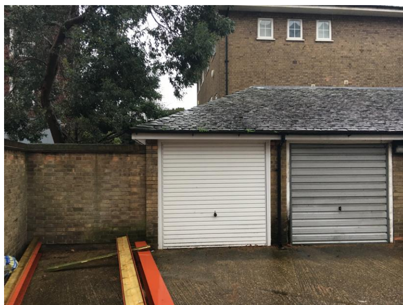
View of Western Elevation
